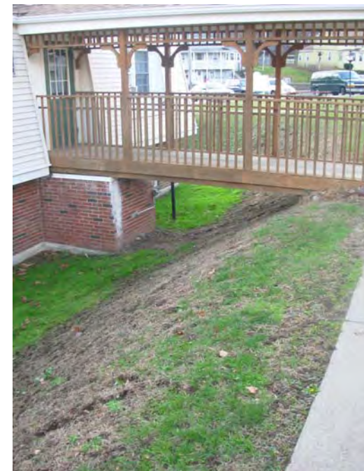
4. Erosion and drainage concerns at hillsides around G.C.E. buildings
