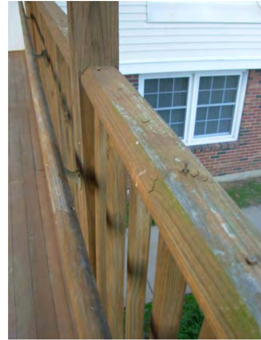
14. Popping nails at some bridge railings a hand hazard
