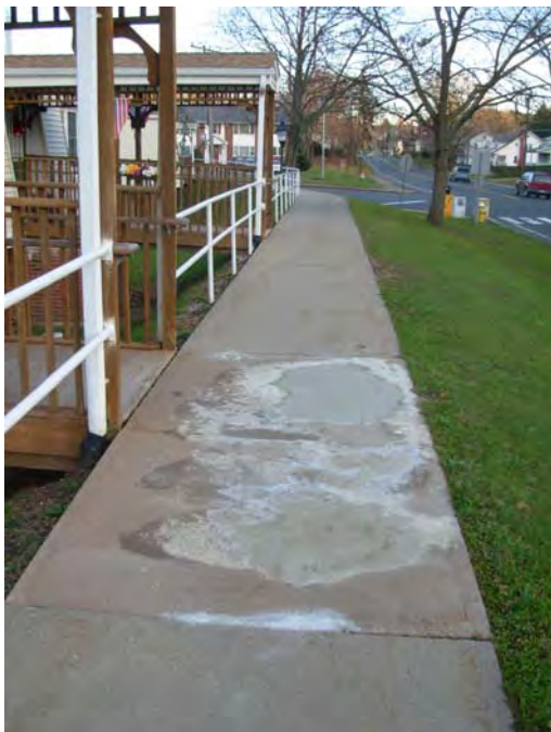
3. Spot concrete walkway spalling and poor repairs
