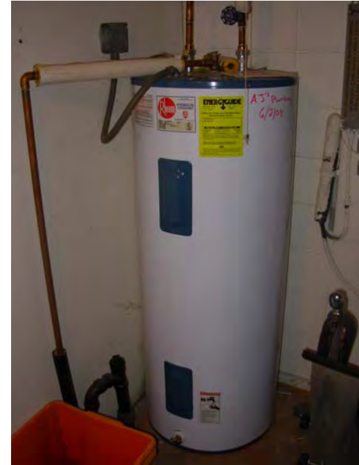
18. DHW serving common area hot water needs
