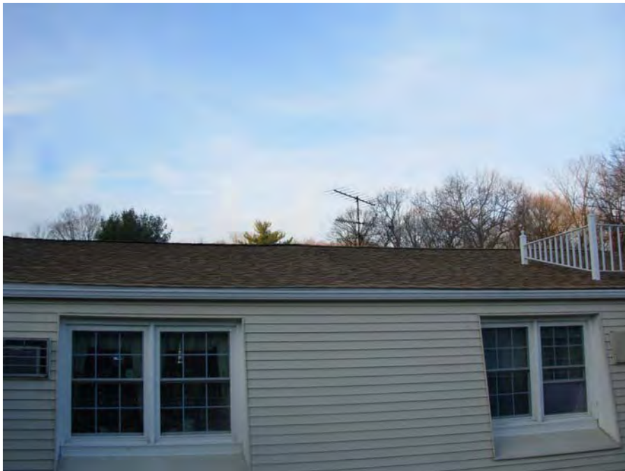
15. Architectural roofing shingles at G.C.E. roofs
