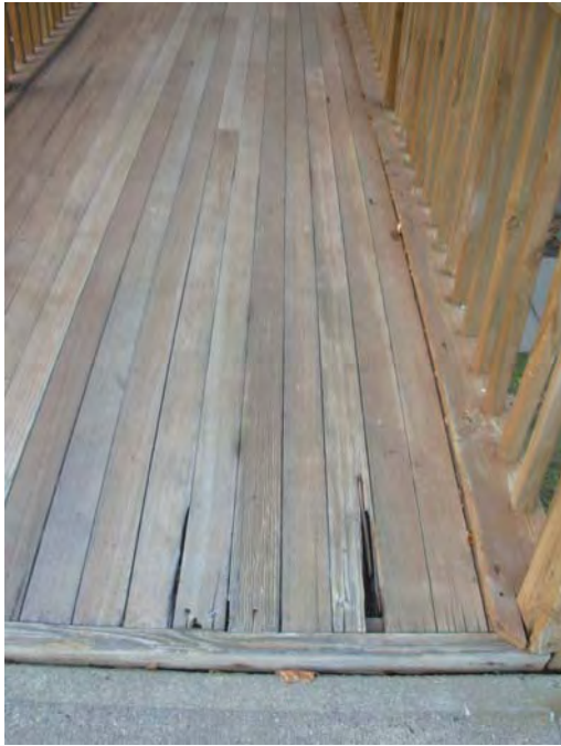
13. Some decking deterioration at bridges
