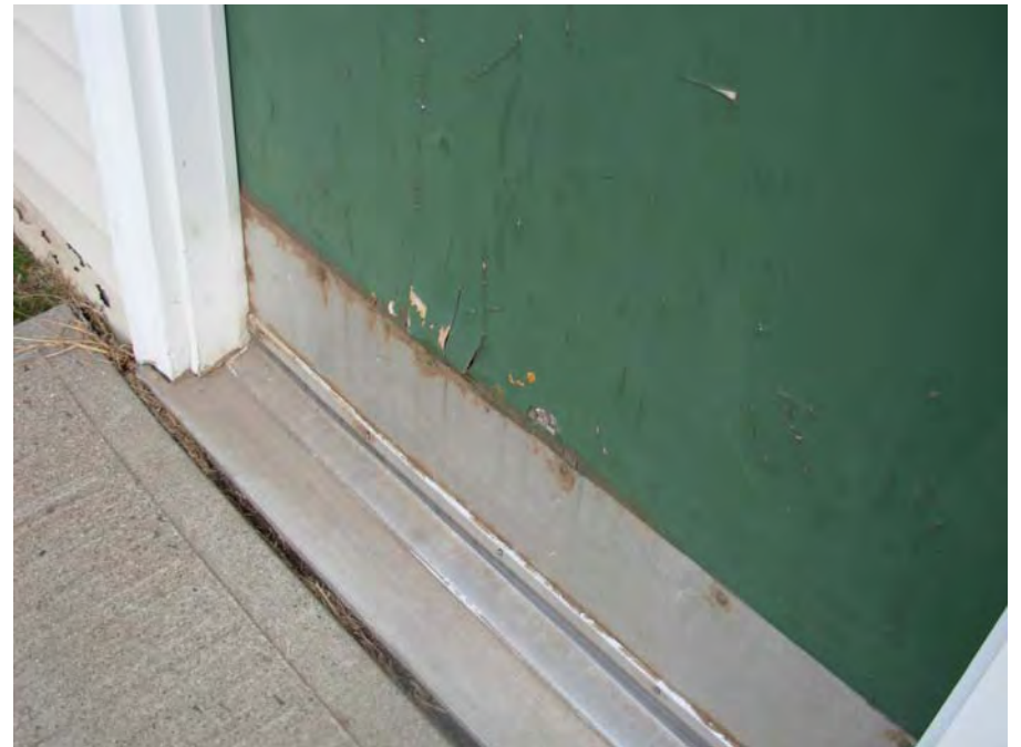
8. Laundry-sitting area doors at G.C. deteriorating
