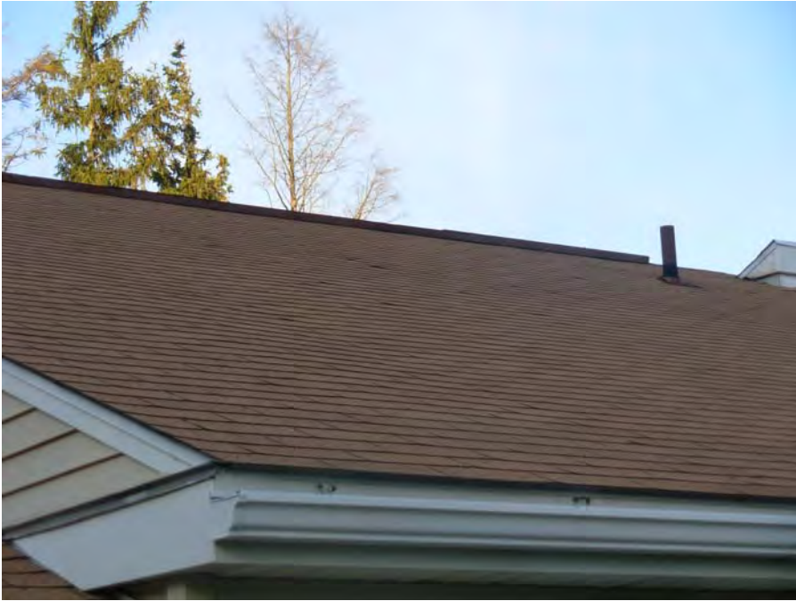
9. Spot lifting of roofing shingles at G.C. buildings
