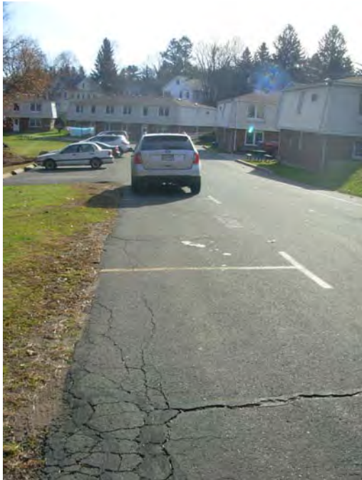
1. Site parking area paving exhibiting some cracking
