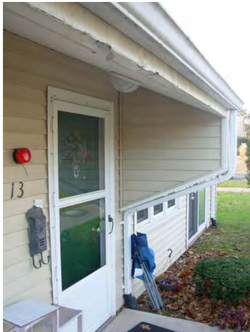
7. Soffit and canopy damage from unit doors at G.C. buildings
