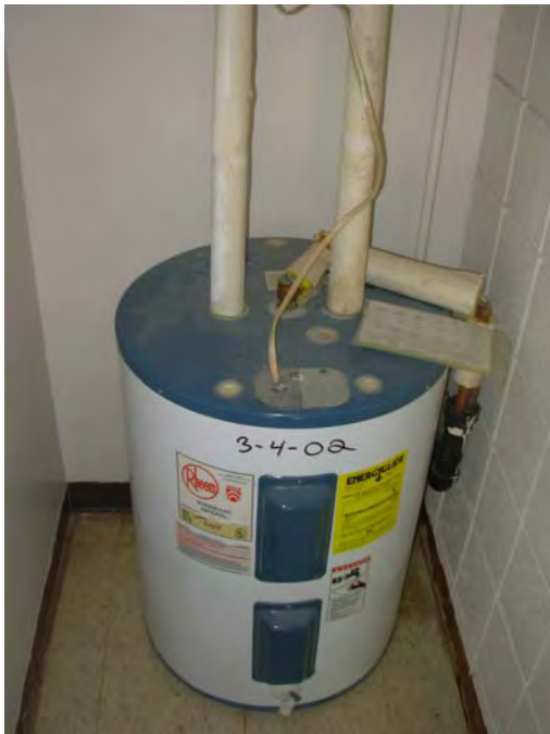
23. Typical unit DHW tank
