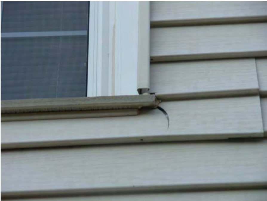
11. Minimal vinyl siding damage observed
