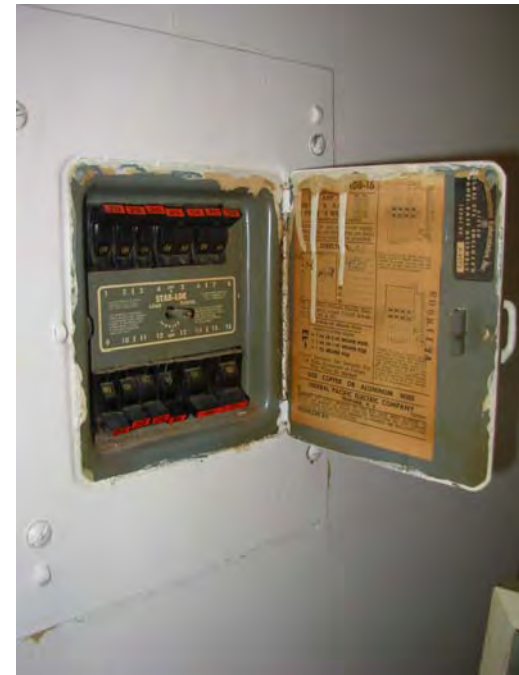
24. Federal Pacific Stablok circuit breaker panels to replace at G.C. units
